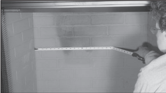
Figure 1 Measure Firebox
